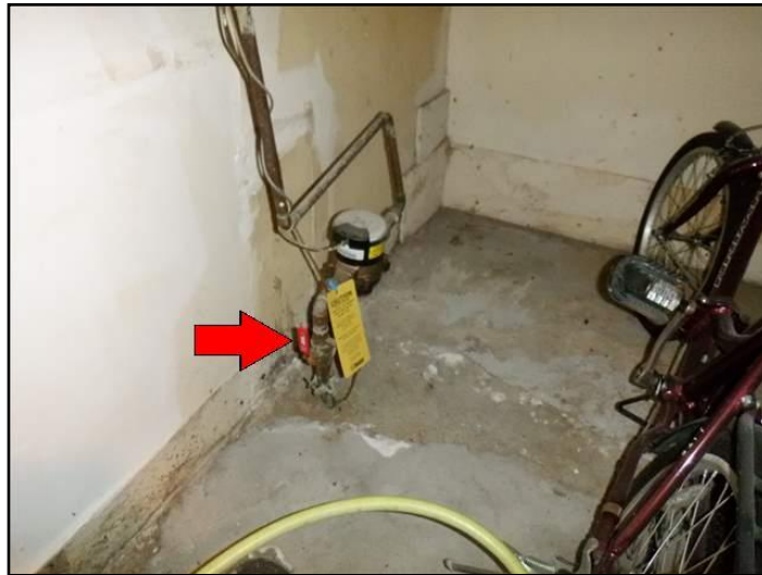
Front of the basement
