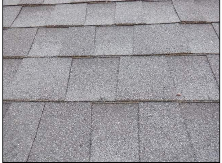
Asphalt shingles
