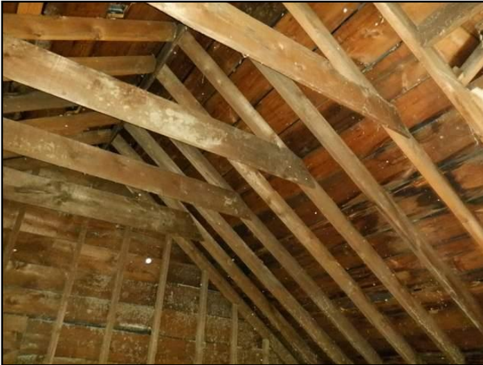
Rafters/roof joists
